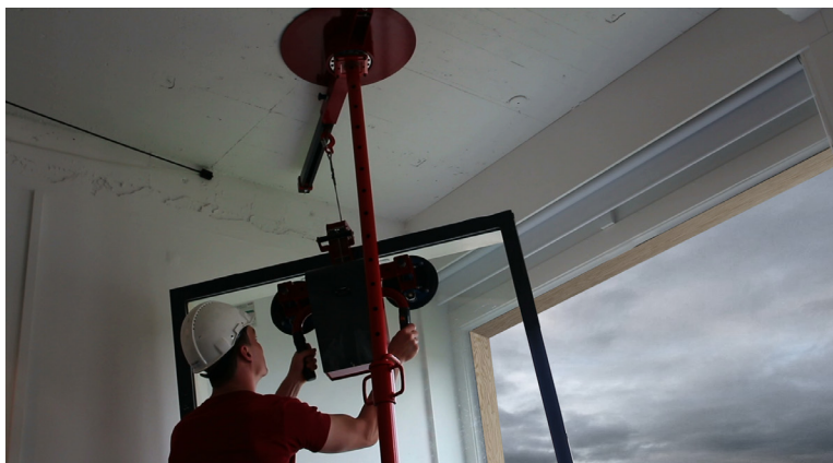
Place and mount window using UPCLIMBER
