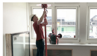
Attach UPCLIMBER and raise column to ceiling
